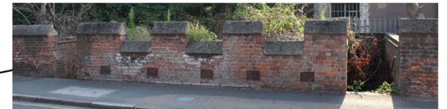
Could the 1899 castellated wall be rebuilt to fit new road alignment? Re-use stone copings.
