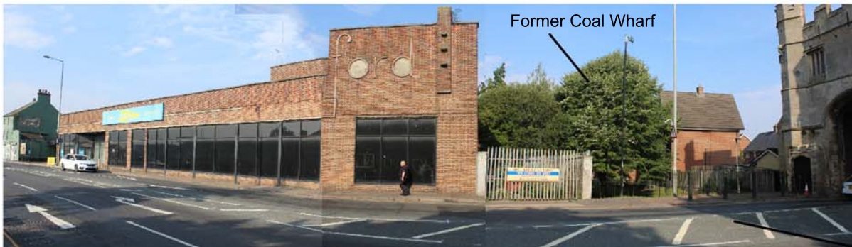
Former Ford garage (Local List). Interesting facade, but little else of sustainable value? Former coal wharf - deserves interpretation and enhancement as amenity area?
