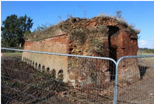
Baines Road brick kiln
